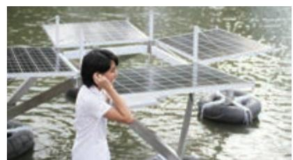
A floating solar power system developed in collaboration with Chulalongkorn University in Thailand. Created by architecture students and others in response to flooding disasters, which occur, without fail, somewhere each year. Specially designed to be an energy station for powering communication devices during a flooding disaster, and subsequently donated to National Science Center for Education in Bangkok.
